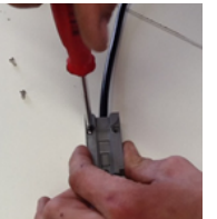
Replace the cut cover and fix it on the terminal with the two screws removed earlier.
